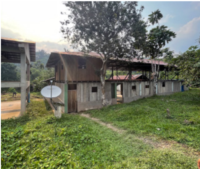
Image 55. ODECOFROC building. View of the building towards the Cenepa River.
